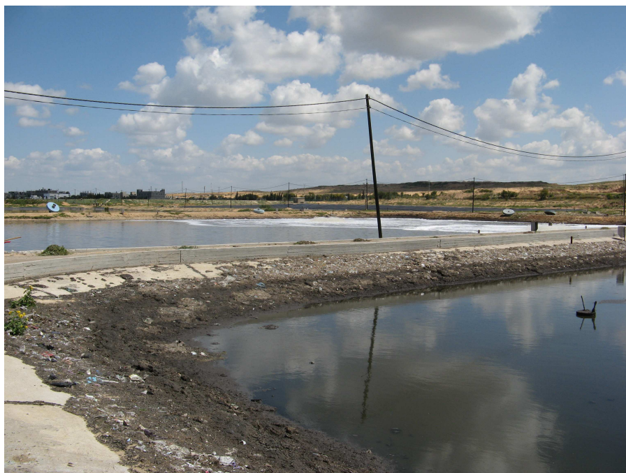
Figure 21 Anaerobic and aerobic ponds, Beit Lahiya Wastewater Treatment Plant, March 2009 (Photograph by Graham Henderson)
