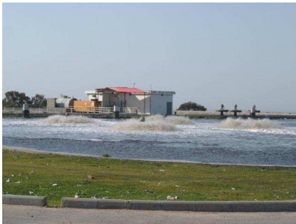
Figure 13 Aerobic pond in Gaza Wastewater Treatment Plant, 2009 (Photograph by Fareed Ashour)
