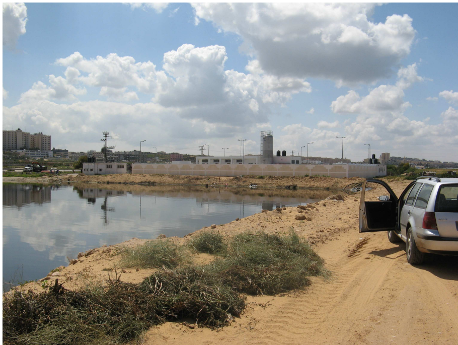
Figure 20 Anaerobic pond and new pumping station, Beit Lahia Wastewater Treatment Plant, March 2009 (Photograph by Graham Henderson)
