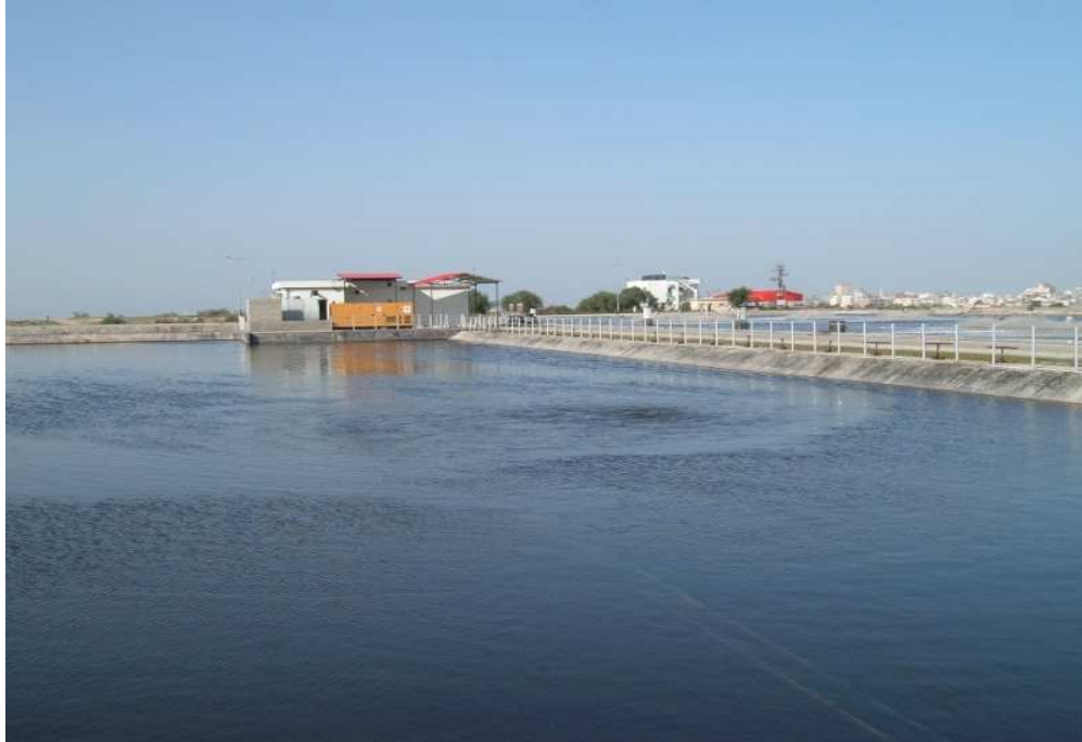
Figure 11 Anaerobic pond in Gaza Wastewater Treatment Plant, 2009 (Photograph by Fareed Ashour)
