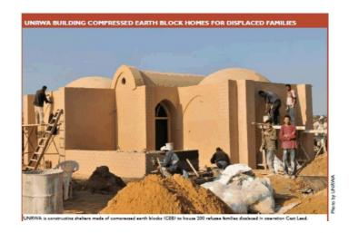
According to UNRWA's latest survey, 200 refugee families are still living in tents or makeshift shelters without proper roofing, windows or doors. In response, UNRWA has launched a project to construct temporary shelters made of compressed earth blocks (CEB). The blocks, made of compressed soil which is plentiful in Gaza and taken from existing quarries, are robust, durable, ecologically friendly and thermally efficient.
