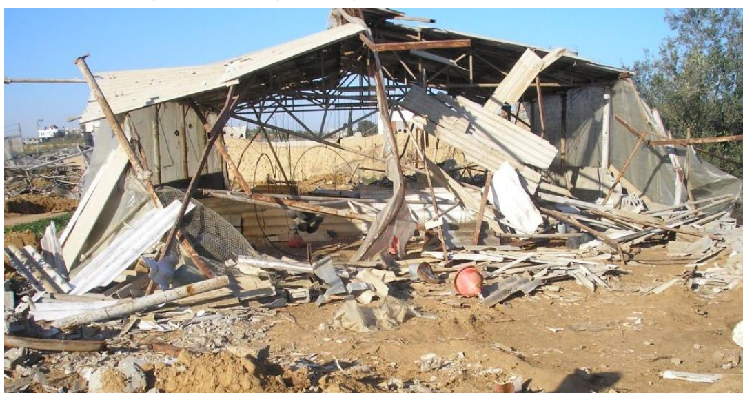
A destroyed agricultural storage building in Al Fukhari
