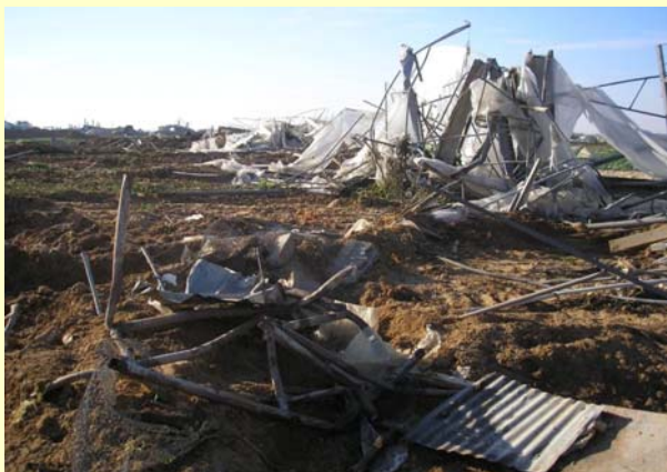
A greenhouse sustains irreparable damage in Al Fukhari
