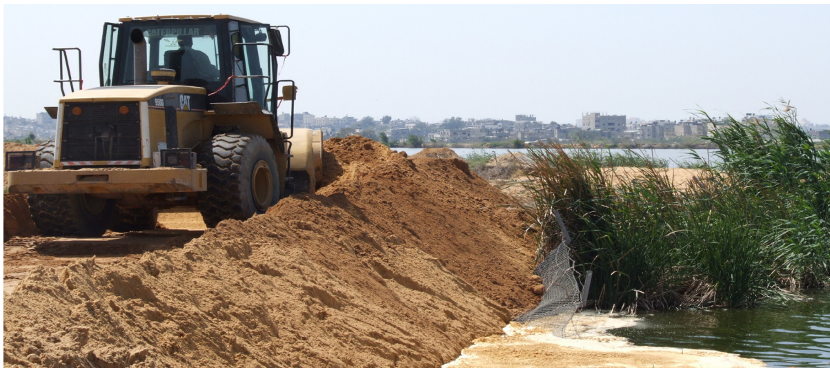
Reinforcing embankment of sewage lake, 1 April 2007 (Source: CMWU)
