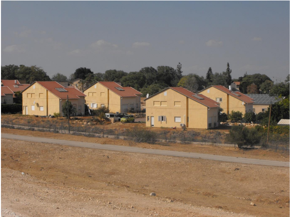
Photo 1: Israeli settlement built environment
