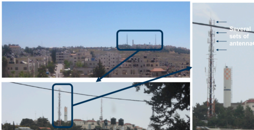
Figure 10: Picture of a mobile tower in the settlement of Psagot
